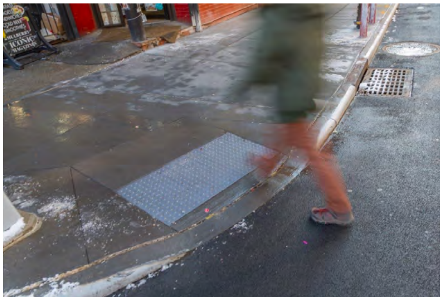
Top image source: Sam Schwartz Consulting. Ann Arbor, MI. Bottom image source: NYC Dept. of Design and Construction.
