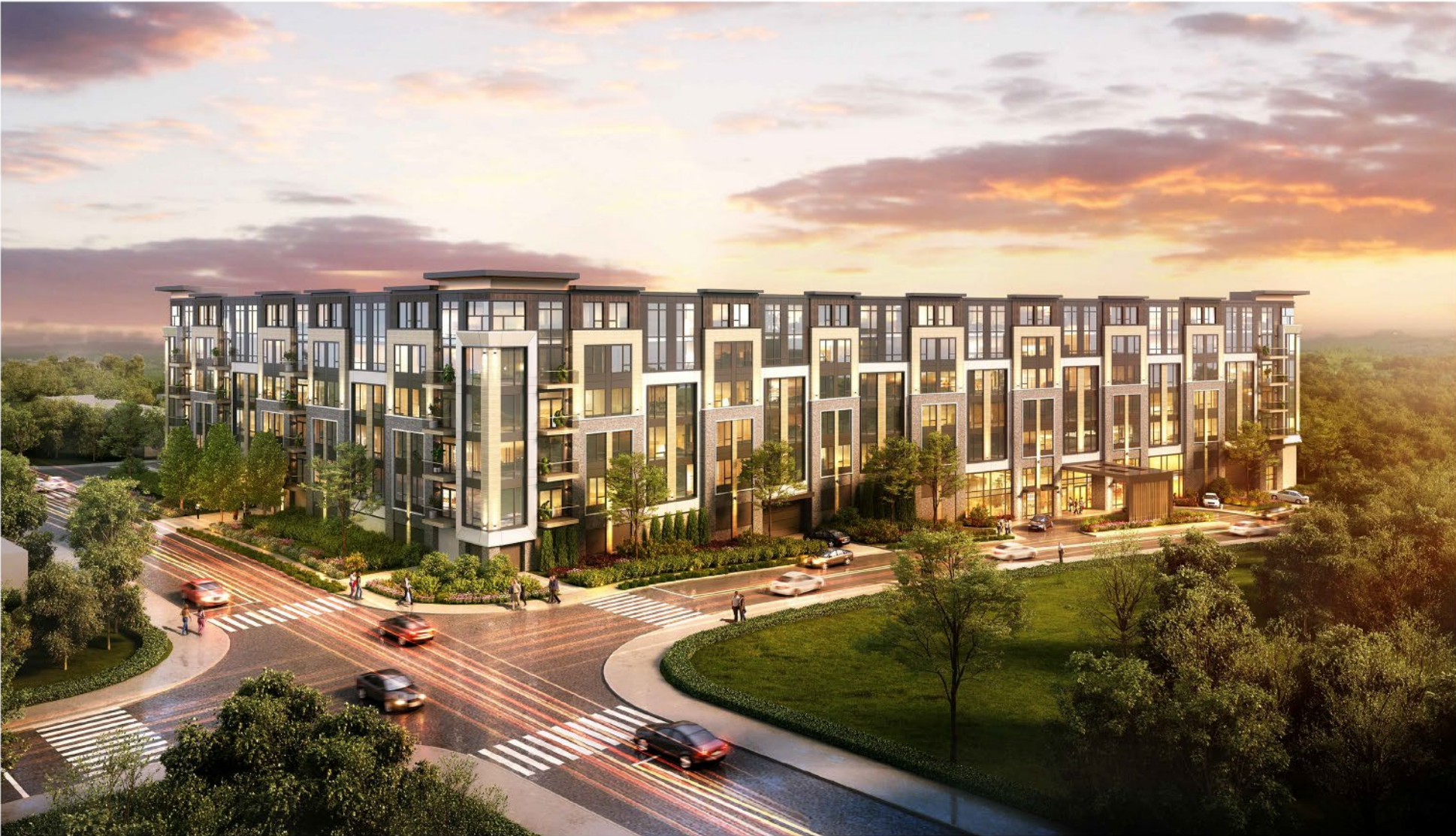
Figure 4: Conceptual Rendering | Redevelopment Plan for 329 Alfred Avenue | Township of Teaneck, NJ PHILLIPS PREISS GRYGIEL LEHENY HUGHES LLC 2020 | Source: CPA Architecture
