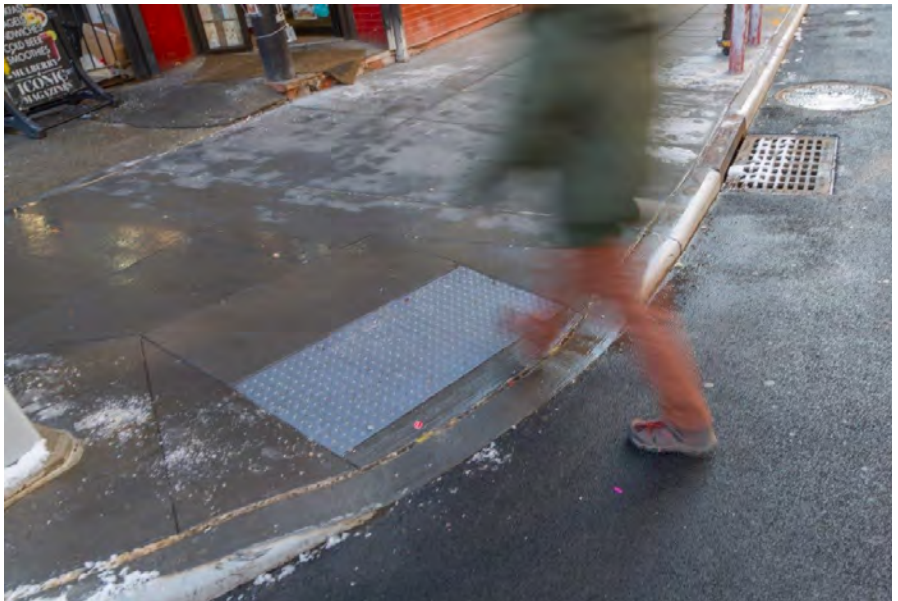
Top image source: Sam Schwartz Consulting. Ann Arbor, MI. Bottom image source: NYC Dept. of Design and Construction.
